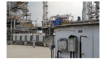
Fertilizer Plant, Bangladesh, AHU
