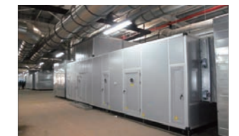
Mercedes Benz Auto factory, Beijing, China, AHU
