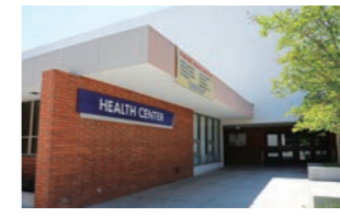
Health Center at Latsia, Cyprus, AHU
